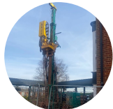
Ground Source Boreholes Drill
