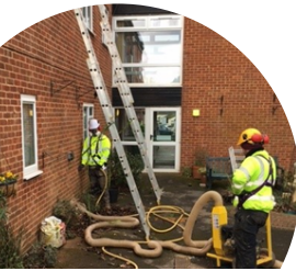
Cavity Wall Insulation
