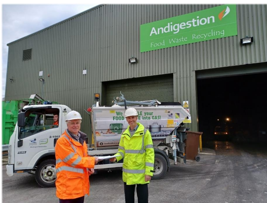
Figure 6 - Andigestion food waste recycling centre
